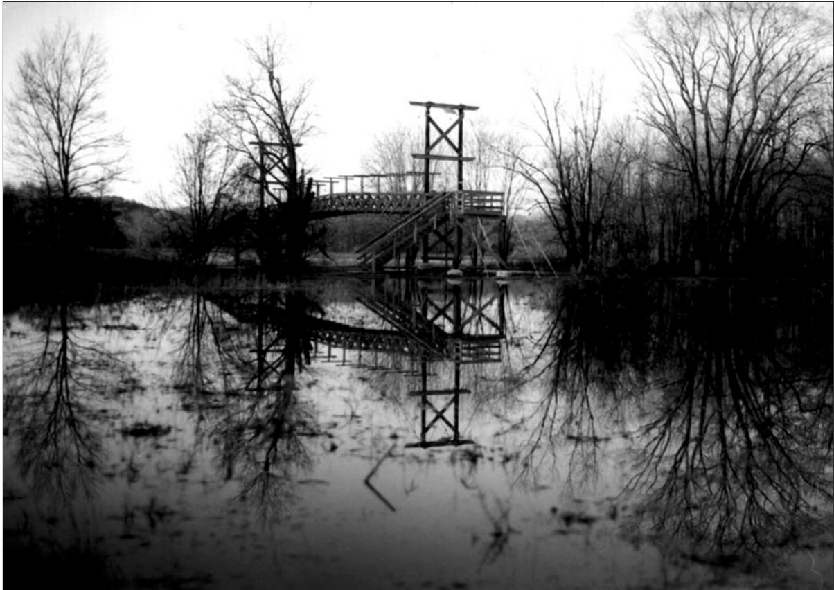
Photo 1a. The Appalachian Trail Pochuck Quagmire Bridge. Photo courtesy of Mr. Stephen Klein, Jr.
